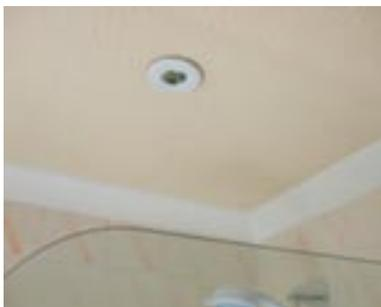
Picture showing a typical IP65 rated downlighter in a zone 1 location above a shower.
