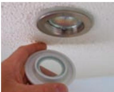
A good quality sealed downlighter, where access to the lamp is gained by simply unscrewing the trim bezel.
