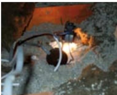
Picture showing poor workmanship at a light fitting.
