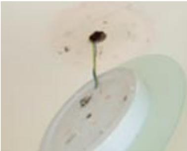
Picture showing a light fitting, with inaccessible connections between the fixed house wiring and the heat resistant wiring tails provided on the fitting.
