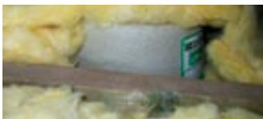
This picture shows a proprietary cover above a recessed downlighter, to allow insulation to be run uninterrupted over it.
