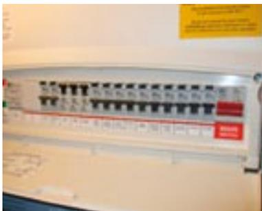
Picture showing BS7671: 2008 compliant consumer unit, with 30mA RCBO protection on majority of circuits – including lighting circuits serving bathroom and shower areas.
