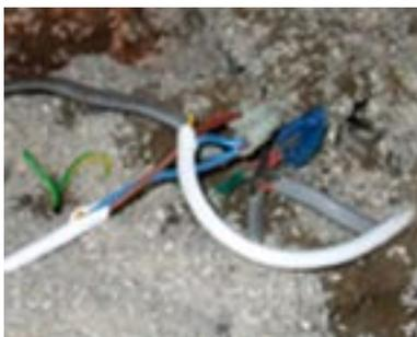
Picture showing poor wiring practice – unenclosed wiring in an attic, following a 2006 bathroom lighting refurbishment.
