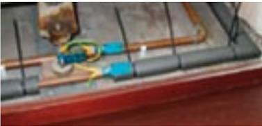
Picture showing supplementary bonding under a bath, which is then linked on to the CPC in the bathroom lighting circuit.
