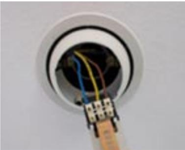
Picture showing a downlighter offering virtually no sound resistance properties.
