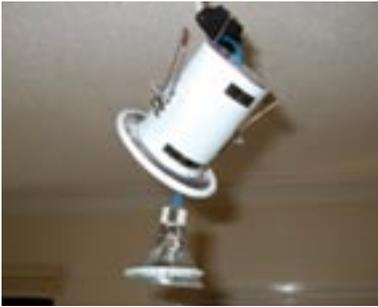
A typical fire-rated light fitting that also meets the requirements for inhibiting moisture passage.
