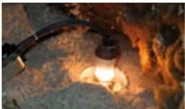
Picture showing the build up of debris behind an open-backed light fitting.
